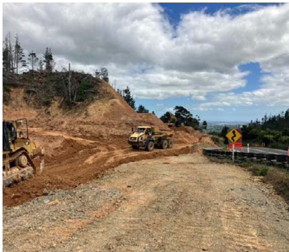
Work on the Brynderwyns - Pic from Waka Kotahi
