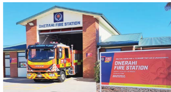
Onerahi Fire Station. Photograph by Nigel Capon
